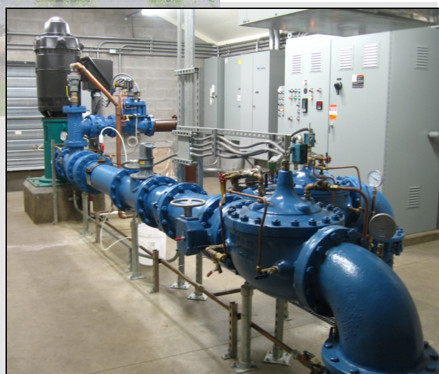
Well No. 5 Pump Motor and Internal Components
